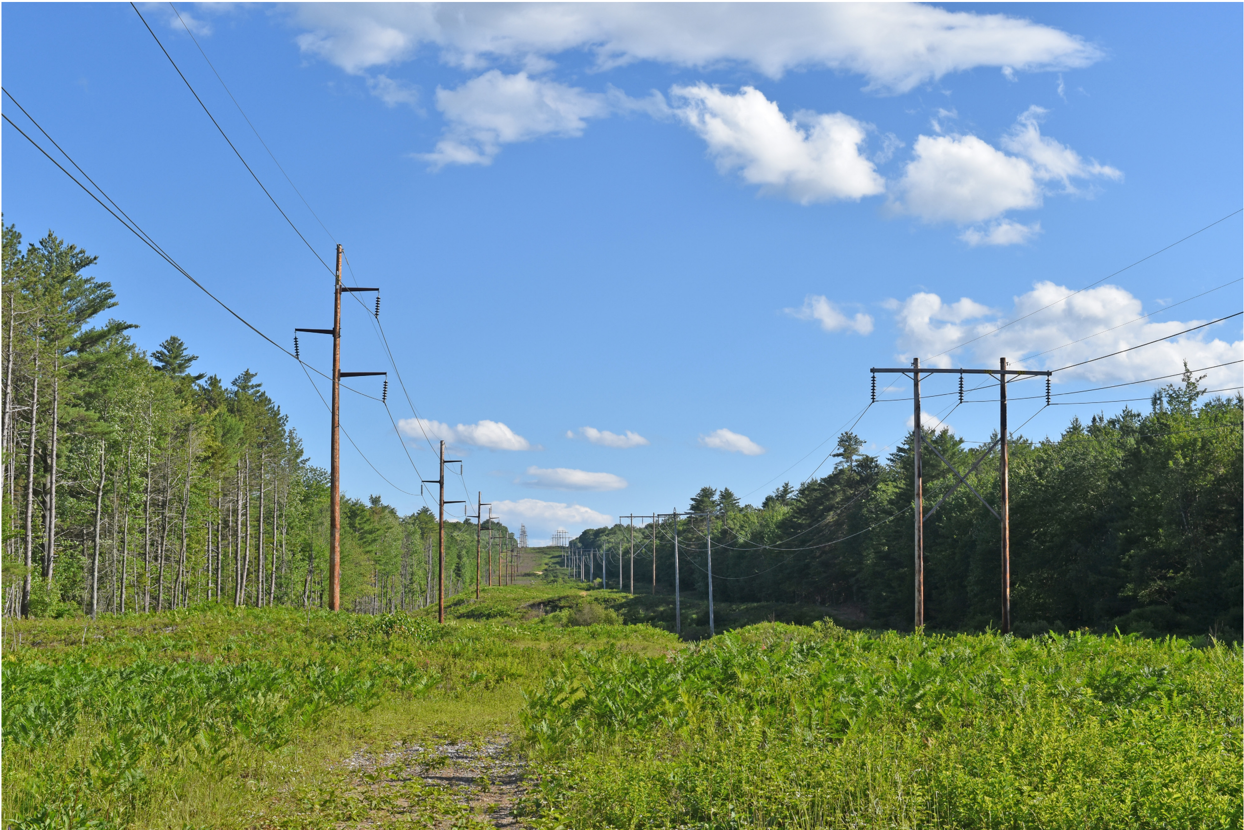
Existing Conditions: Normal view looking south from an access road within the Androscoggin Riverlands State Park crossing the existing transmission line.
