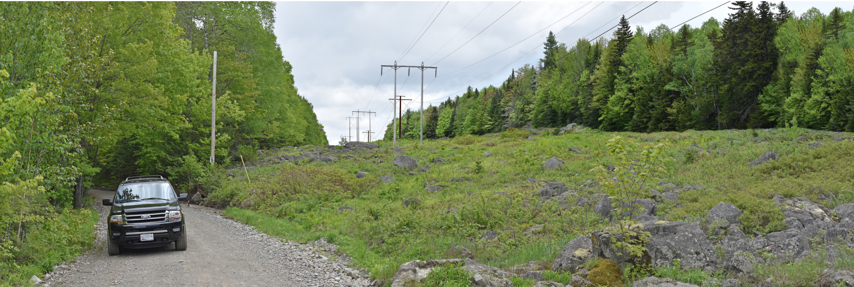
Proposed Conditions: Panoramic view looking southeast to south from Troutdale Road in The Forks Plt. toward the proposed co-located HVDC transmission line. Troutdale Road is located within the existing 115 kV transmission line corridor for approximately 1,000 feet. The existing 150’ wide corridor clearing will be widened by 75’ on the western side to accommodate the new transmission line. Two HVDC transmission structures will be visible looking to the southeast, and four looking to the northwest. See Appendix B: Study Area Photographs for additional images.
