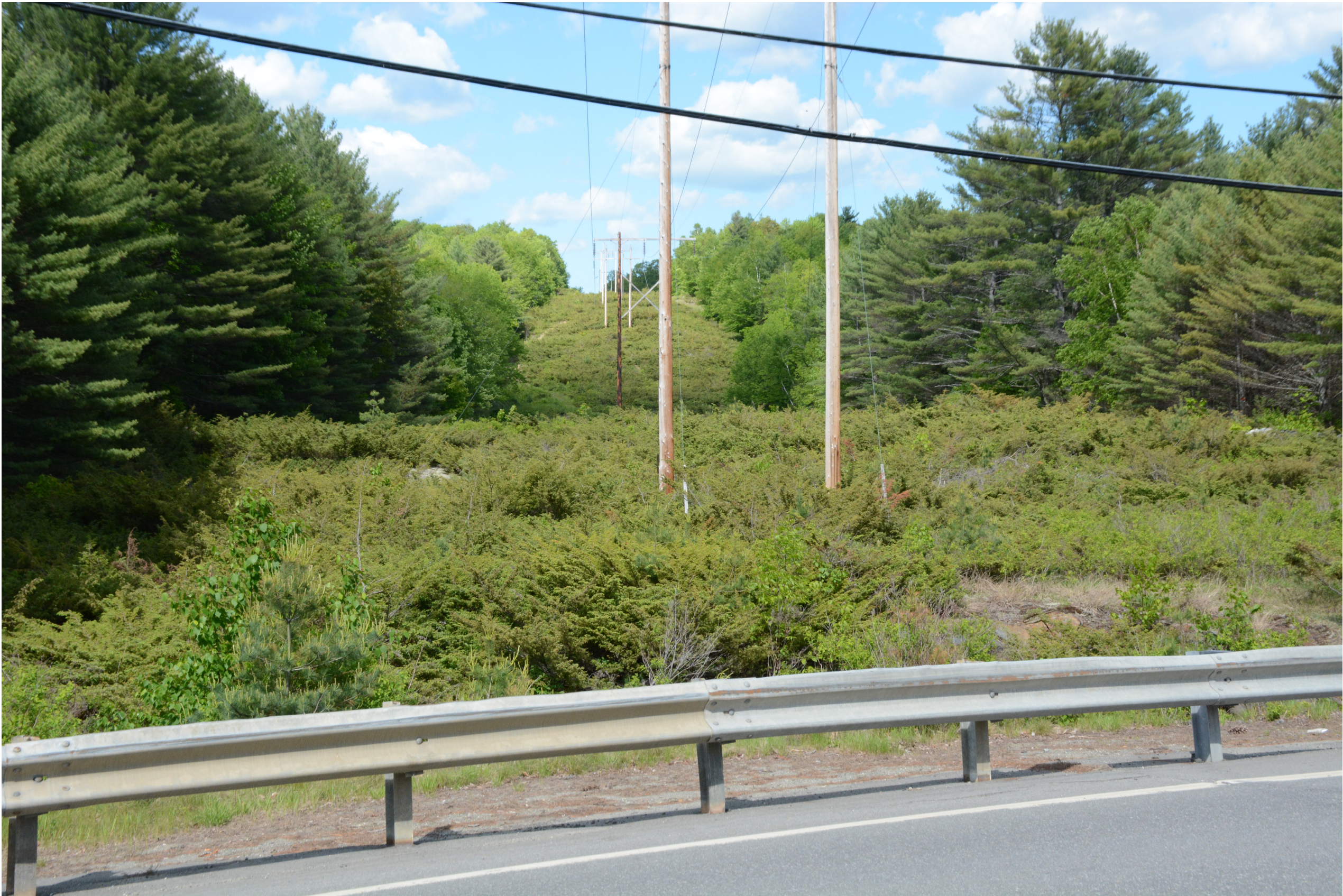
Existing Conditions: Normal view looking east from Route 201 toward the existing 115 kV transmission line corridor.
