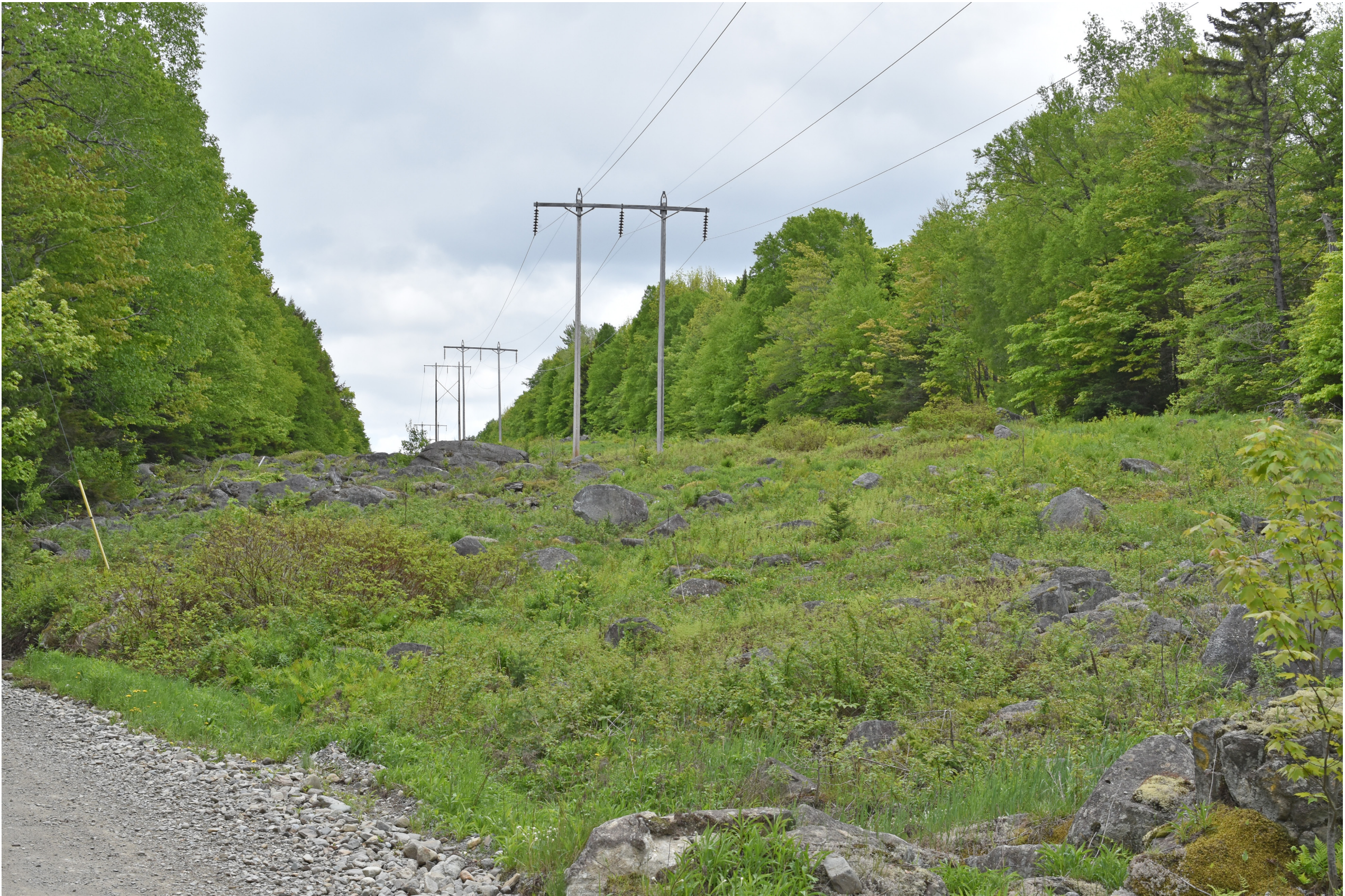
Existing Conditions: Normal view looking southeast from Troutdale Road toward the existing 115 kV transmission line within a 150’ wide cleared corridor.
