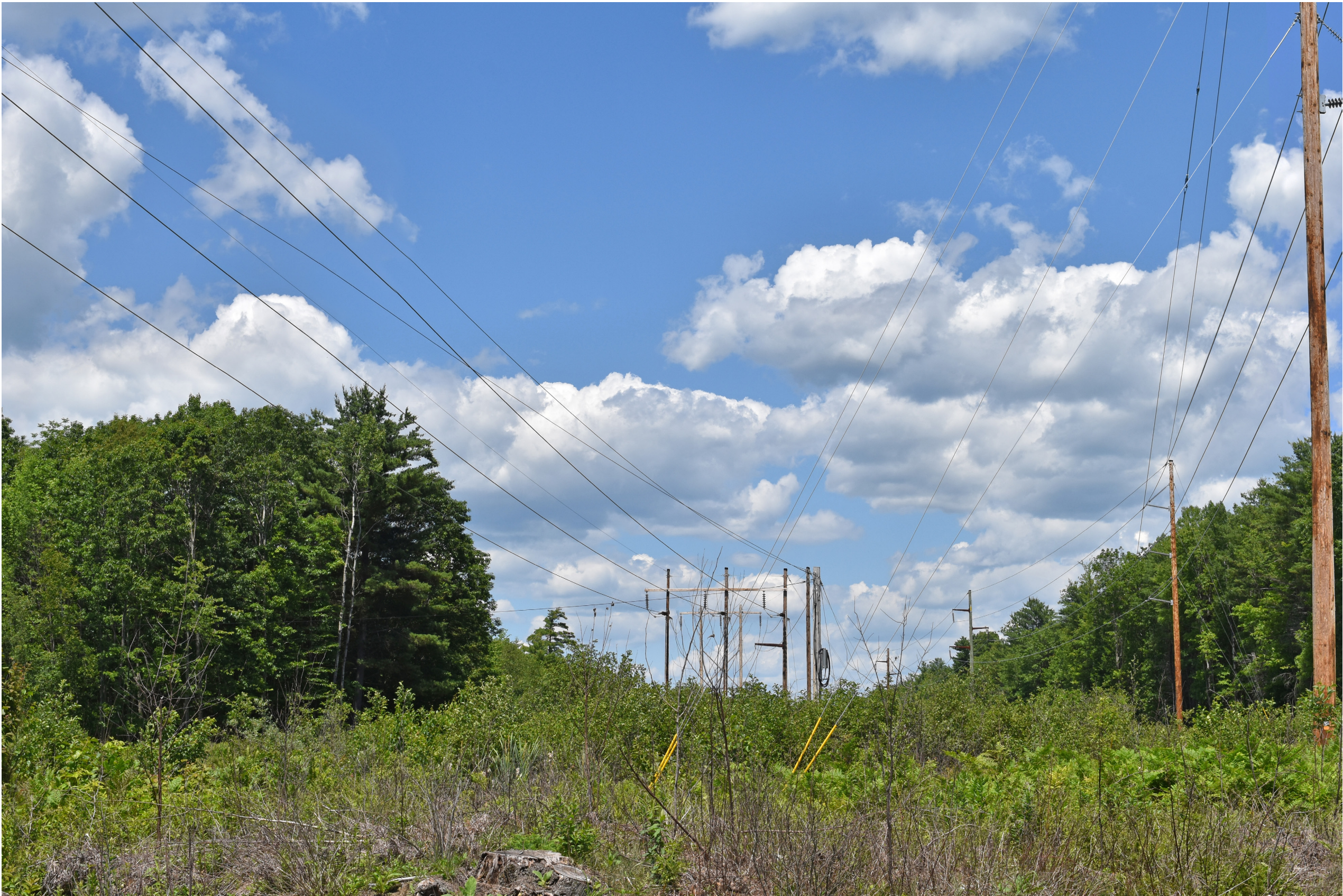
Existing Conditions: Normal view looking from north from Merrill Road.
