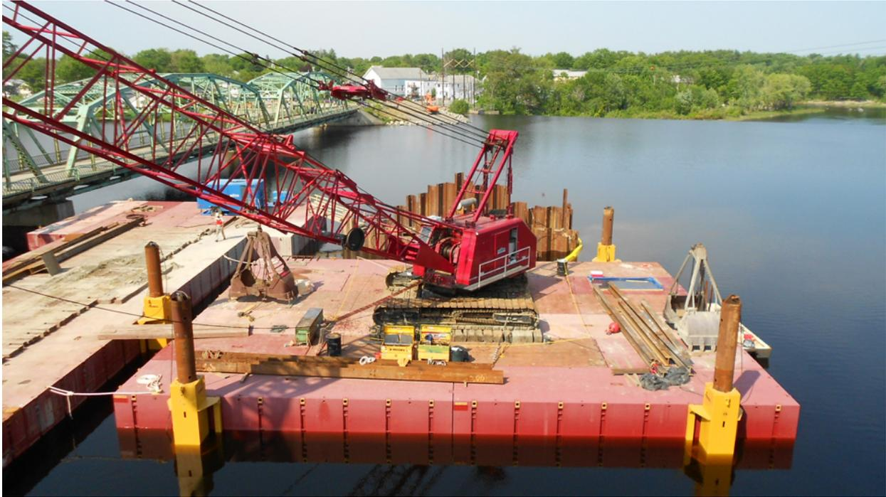
Example of a spud barge with crane, clamshell suited for this work.
