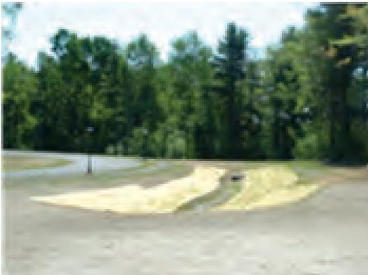
Vegetated swales need to be stabilized early during the growing season (by September 15) or protected with an erosion control blanket or riprap.
