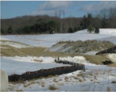
Stabilization during the winter construction period may include mulching, erosion control mix, erosion control blankets, and stone.
