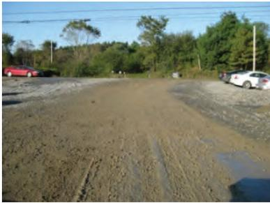
The pad should be inspected weekly as well as before and after a storm. The pad may have to be replaced if the voids become filled with sediment. Street sweeping may be necessary.
