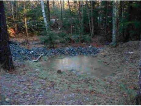
Typically, a level spreader should be no smaller than 12 feet.
