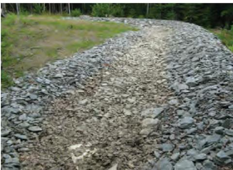
The length of a level spreader should be based on the expected runoff volume and slope of the receiving buffer.
