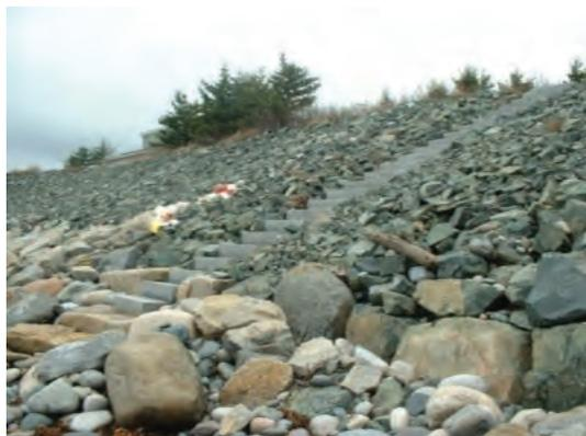
Slopes steeper than 1.5:1 or longer than 6 feet should be engineered.
