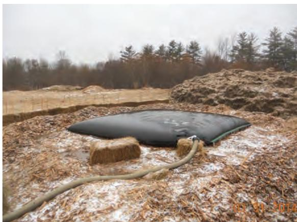
Filter bags have a finite capacity for sediment collection and may be prone to plugging. Avoid over-pressurizing the bag or it may burst.
