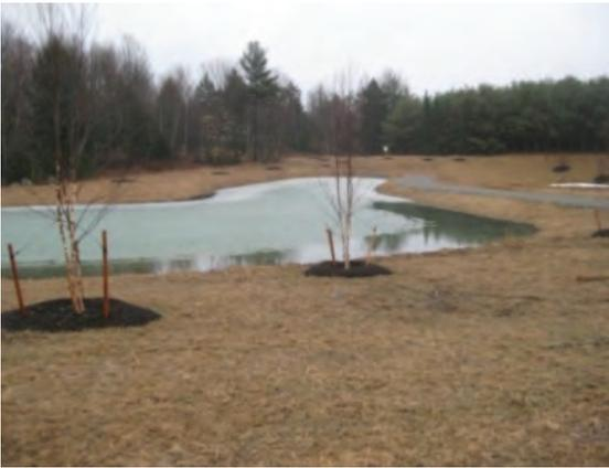
A mulch cover should be heavy enough to resist disturbance or should be anchored. It will last only 2-3 months and may need to be reapplied if grass growth is inadequate.
