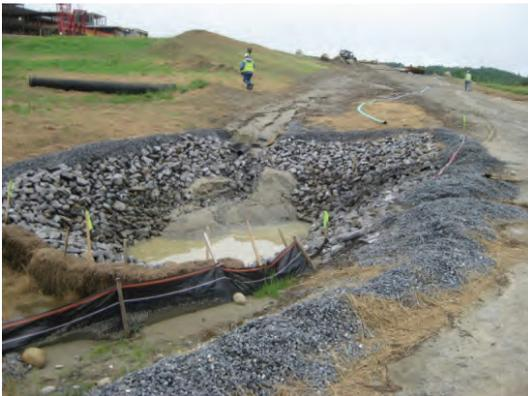
Remove sediments when accumulation reaches the mid-point depth of the trap.
