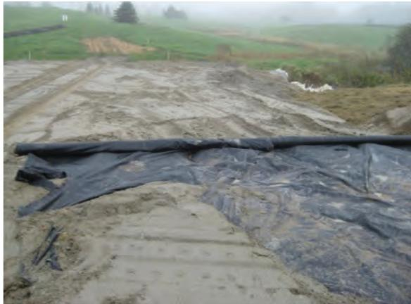
**WOVEN GEOTEXTILES** are mostly used for soil reinforcement beneath sharp, angular aggregates if dropped more than 5 feet; and where the cover will be more than 10 feet thick. It may be used for seepage management if the fabric's openings are smaller than the soil gradation. A woven filter fabric is usually used in a road base to provide bearing capacity and linear strength over a soft subsoil.
