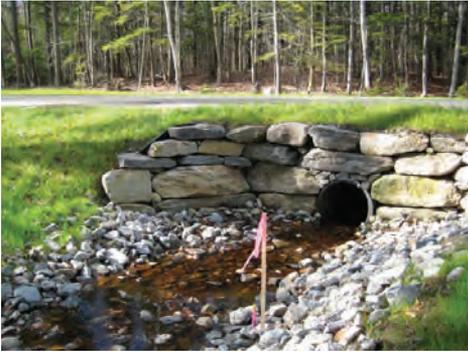
After installation, the streambed should be restored to its original shape and slope.
