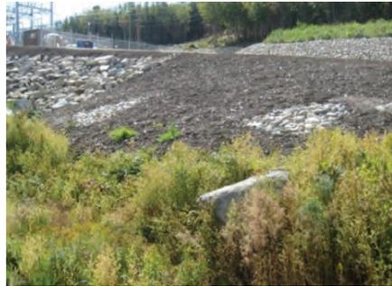
Regularly inspect the slope and after severe storms for slumping, sliding, or seepage problems. The sides of the riprapped area may be prone to instability or erosion. Correct any problem immediately.
