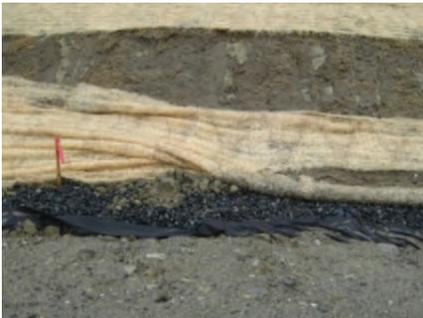
A continuous contact between the mat and the soil is critical, otherwise the mat may fail.
