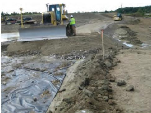
**GEOTEXTILE FABRIC** will strengthen the road when constructed over soft or poorly drained underlying soils that are prone to tire rutting. A woven geotextile will provide linear strength by distributing the vehicle weight over a broad area.
