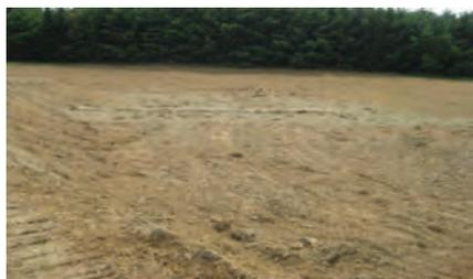
Newly seeded beds should be inspected regularly. Any sign of rill or gully erosion should be repaired as soon as possible.
