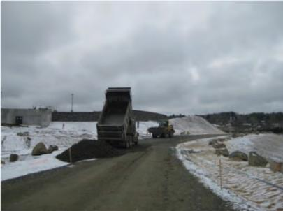
The preferred road construction is above natural ground elevation for positive drainage. Cuts and fills are more of the norm for roads constructed along the contour of sloping sites.
