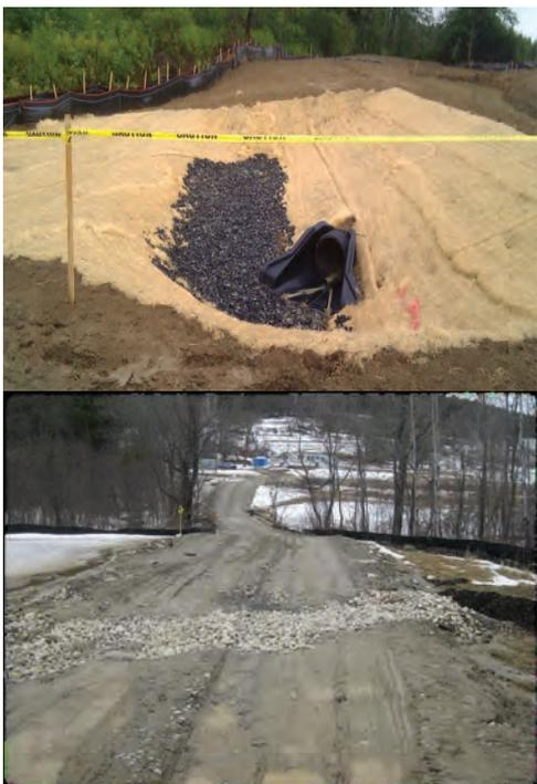
**WATERBARS** are constructed at a 30-45 degree angle to intercept and direct runoff out of the travel way and for dissipation to the side. Waterbars should be spaced every 250 feet on a 2% road and every 30-40 feet for roads with a 20% grade. In bends or where surface runoff needs shed to one side, the road may be super-elevated. Broad-based dips have a wider base than waterbars and are more appropriate on year-round roads.
