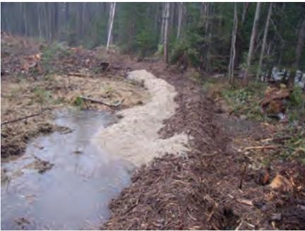
The spreader should be level and prevent channelization. In a temporary situation, erosion control mix or a berm of brush may provide the velocity reduction necessary to promote dispersion.
