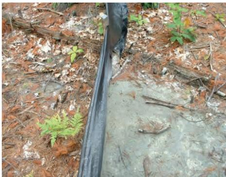
Collected sediments should be removed when one-half the height of the barrier is filled.
