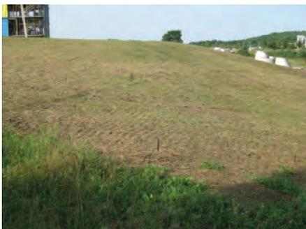
Inspect periodically the re-vegetated area. To be considered stabilized, 95% of the soil surface should be vegetated or the area may need reseeding and mulching.
