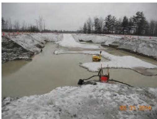
The water removed from the excavation area should either be discharged as sheet flow to a buffer area or to a treatment structure.
