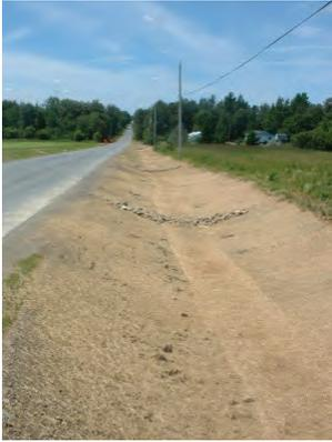
During construction inspect the channel daily and during storm events to check for erosion. Repair as needed. After the channel is stabilized, maintain a channel that is stable and free of debris.
