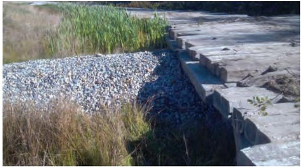
**SURFACE FLOW DIVERTED BY A SWALE**
