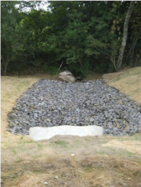
The riprap should extend across the bottom and up both banks of the channel to the maximum height of flow or to a point where vegetation can be established.
