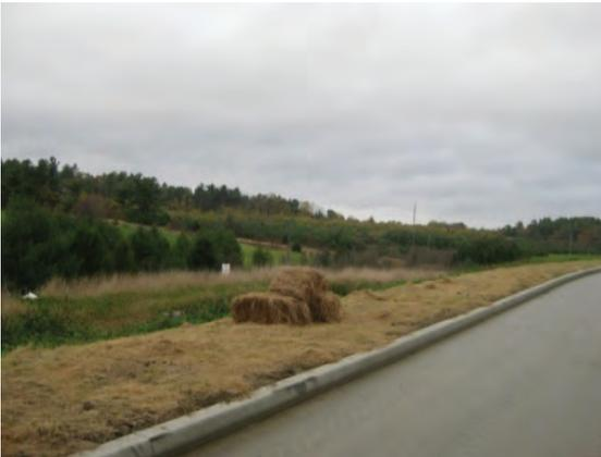
Areas which cannot be revegetated before winter must be mulched at the winter rate with double the mulch and with dormant seeding for spring growth if the site is ready to be permanently stabilized.
