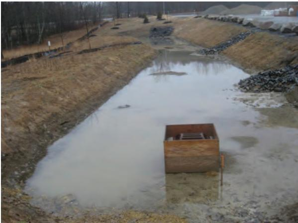
An emergency spillway is necessary unless a piped outlet can pass all peak flows without overtopping the embankment.
