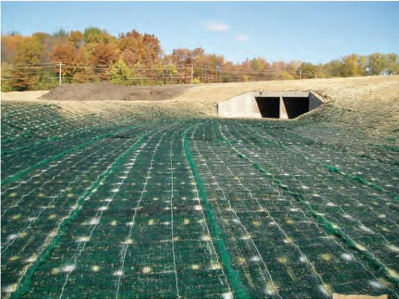
Inspect the area for erosion and repair immediately until vegetation has a full catch of grass (95%).
