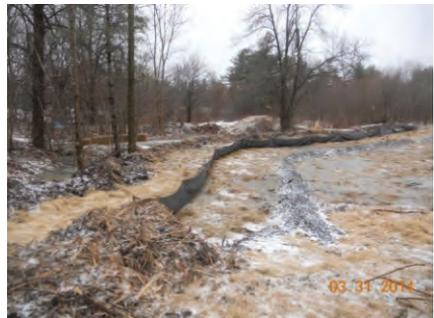
Sediment barriers should be inspected and repaired before, during, and after each rain event.
