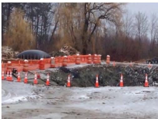
During dewatering, frequently inspect the receiving area for signs of erosion, concentrated flows or sediment discharge and repair immediately.
