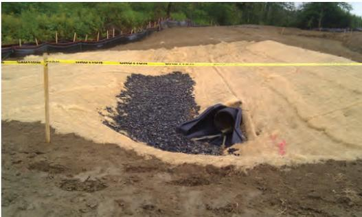
An erosion control blanket is recommended to protect new seeds from washouts. Install per the manufacturer's specifications.
