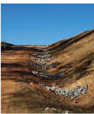
Any erosion downgradient or around the edges of stone check dams should be corrected immediately.
