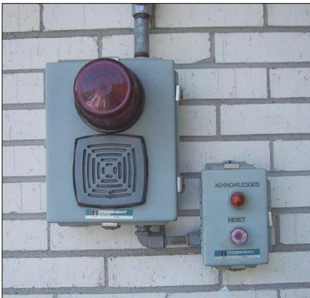
*This is a typical unlabeled overfill alarm. These alarms should be labeled so the delivery driver knows where it is and what it is.*
