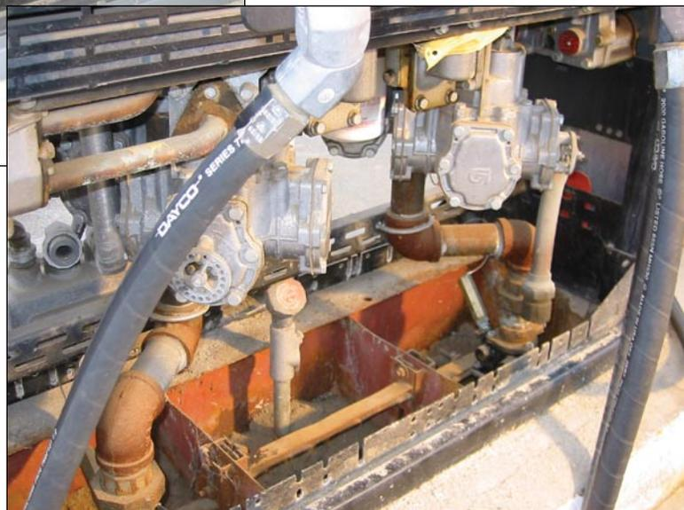
*If a dispenser has no containment sump, leakage from any of the dispenser components goes directly into the ground. If the leakage goes undetected, serious contamination problems can result.*
