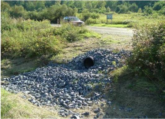
*Stabilizing culverts and maintaining roadside ditches can help reduce erosion and sedimentation.*
