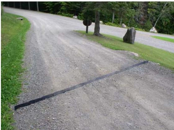
*Example of a rubber water diverter used to prevent erosion on State Park roads.*
