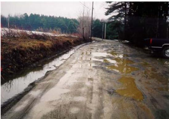
*Poorly maintained roads and ditches provide direct conduits for phosphorus laden sediment to Echo Lake (Bordner 2001).*
